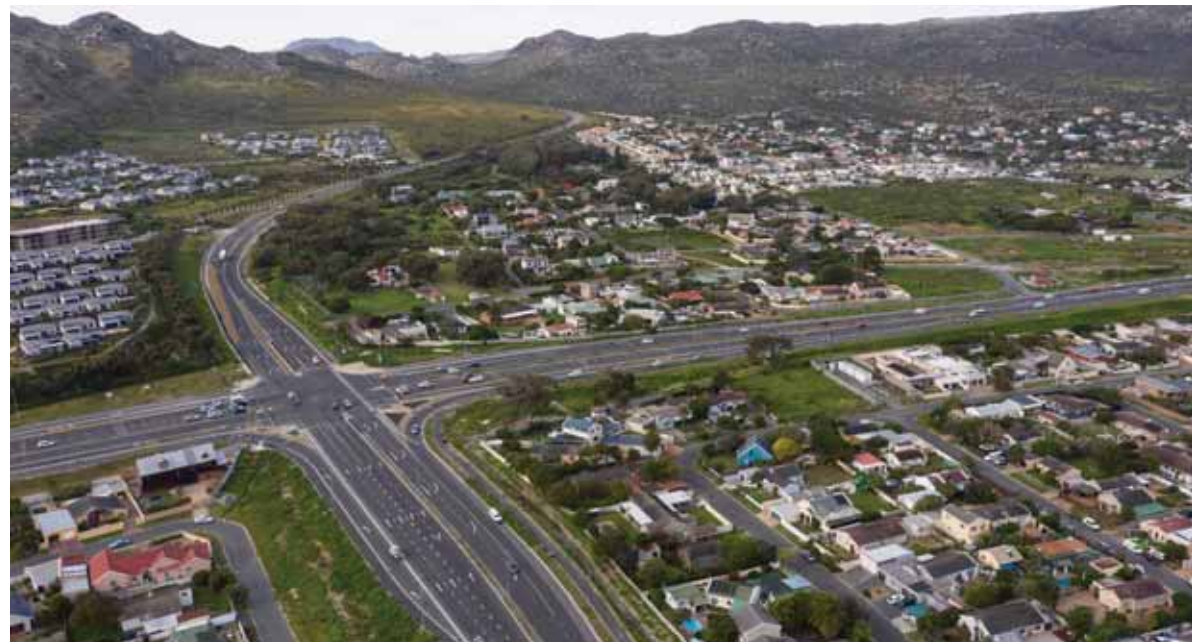
The time has 'Kommetjie': The recently completed R256 million, four-year Kommetjie Road congestion management project entailed roadworks of approximately 3,5 km and the creation of safe facilities for pedestrians and cyclists.
